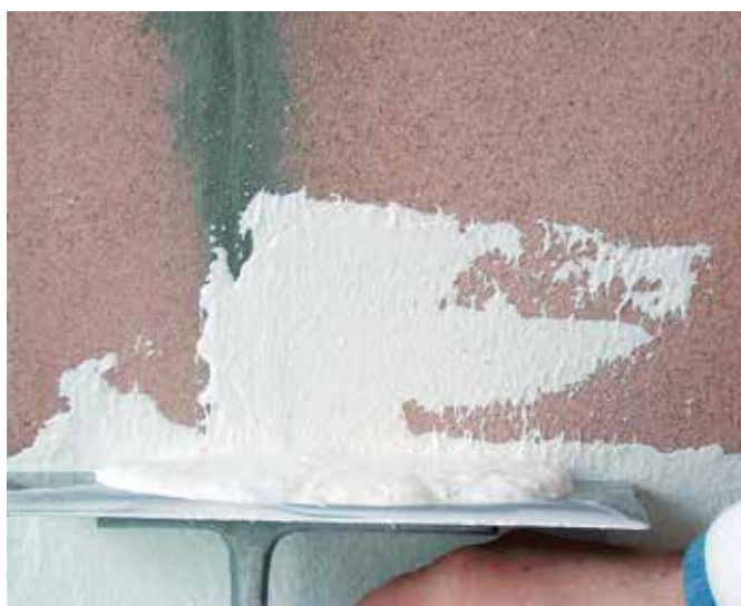
4 | Total leveling treatment with a coat of raselast
