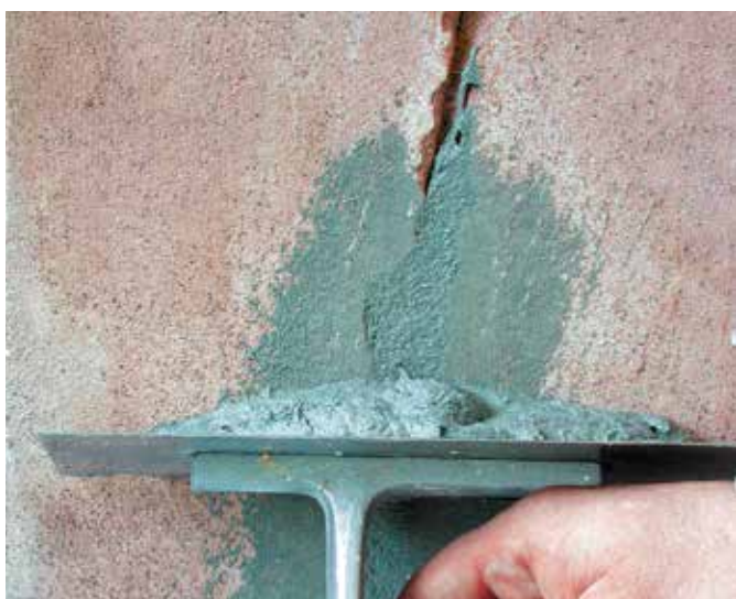
3 | Sealing the crack with raselast mixed with cement
