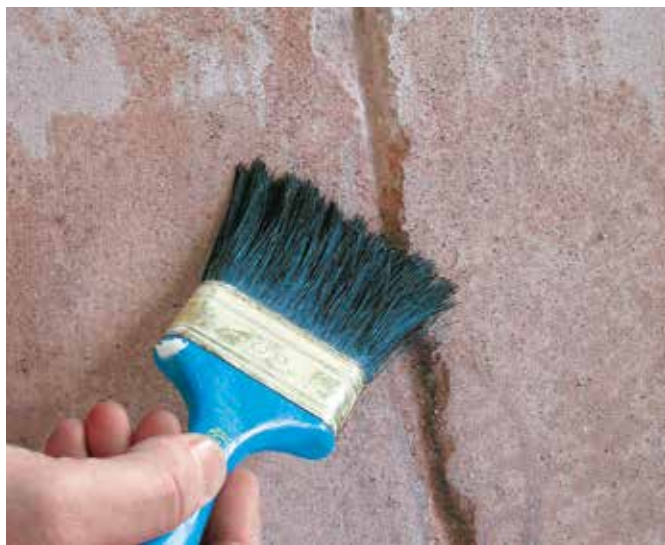
2 | Application of primer (interior walls) or stabilizer (exterior walls)
