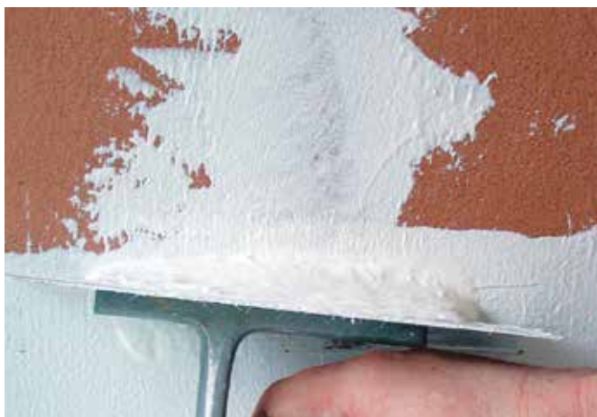
3 | Leveling with raselast
