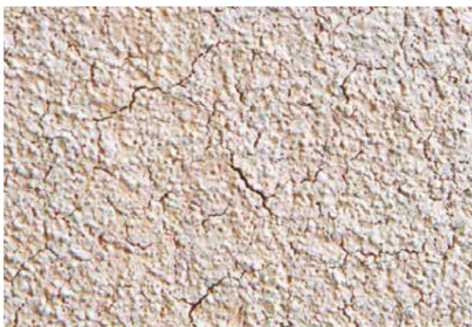
1 | A dry and clean cracked surface
