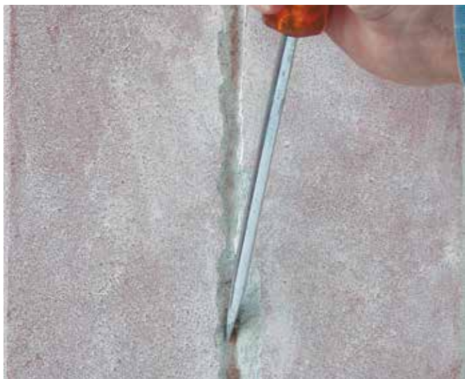
1 | Expanding the crack
