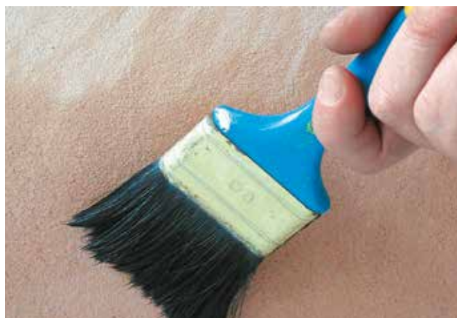
2 | Application of primer (interior walls) or stabilizer (exterior walls)
