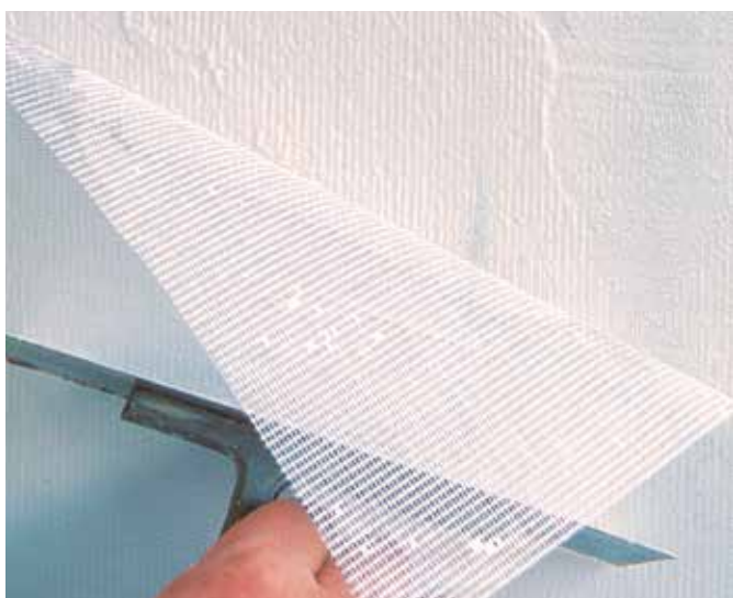
5 | Application of fibralarge and leveling treatment with second coat of raselast
