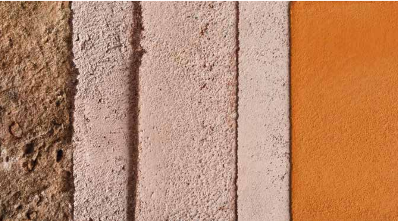
Facade stratigraphy composed of: stone structure, render in rialto malta grezza blended with cocciopesto powder, layer of malta grezza blended with cocciopesto , malta fine blended with cocciopesto , rialto antiqua 1 finish.
