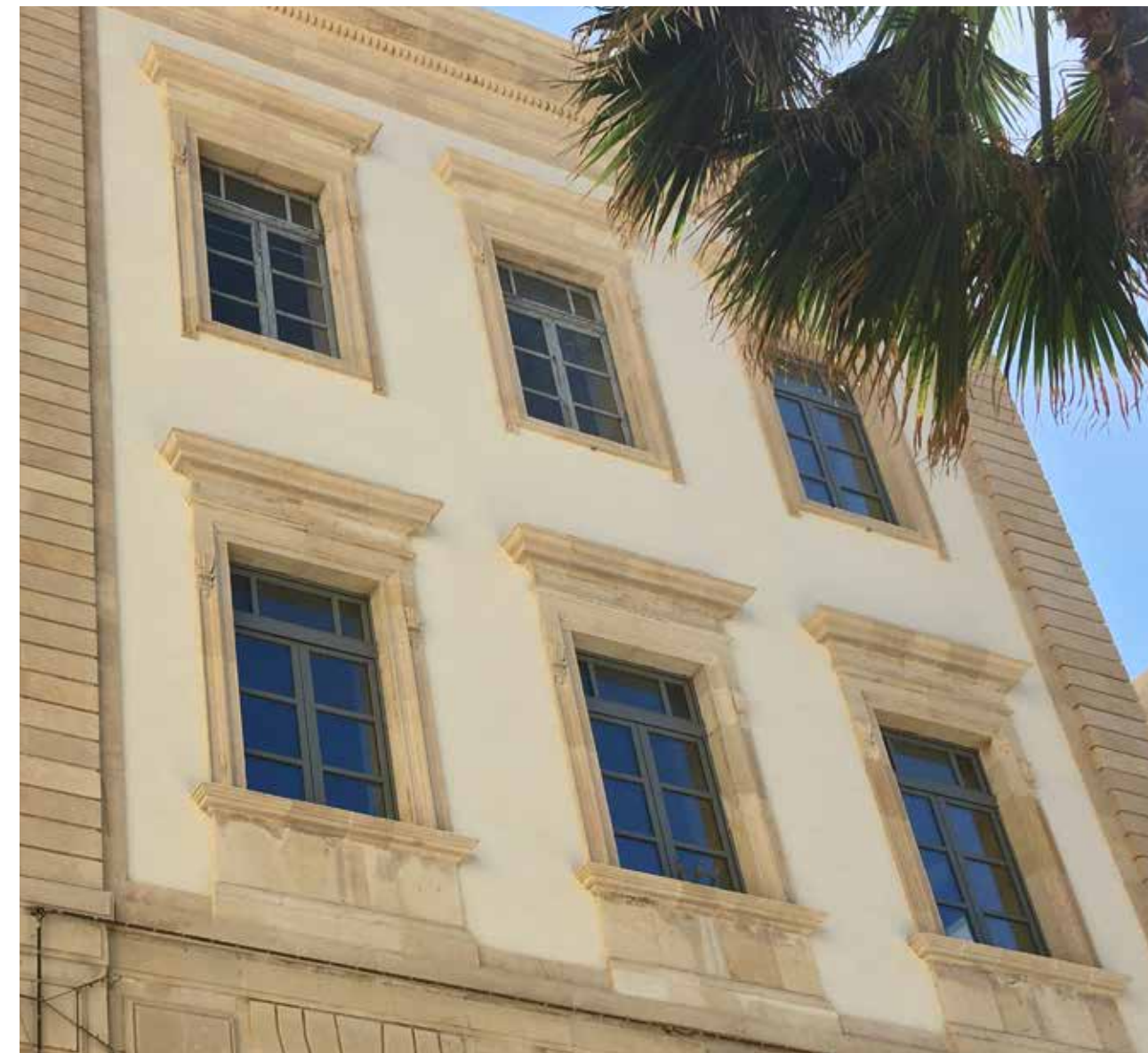
rialto antiqua 1 sponge trowel "frattazzato" effect color 019 berenice from the rialto "CENTO COLORI" color chart for lime plaster
