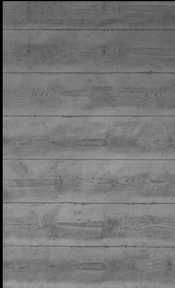
formwork concrete: application with a stainless steel trowel and wood graining rubber tool color s346
