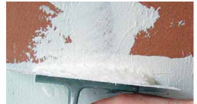
(3) Leveling with rialto raselast
