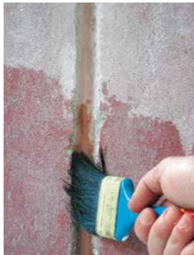
(2) Application of rialto primer (interior walls) or rialto stabilizer (exterior walls)
