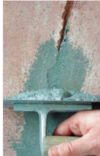
(3) Sealing the crack with rialto raselast mixed with cement
