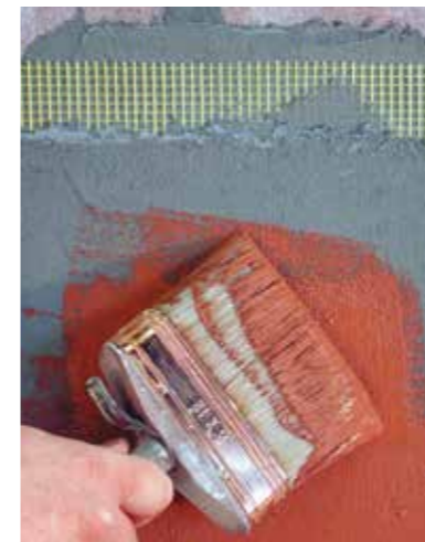
(6) Application of rialto finish or rialto domosil
