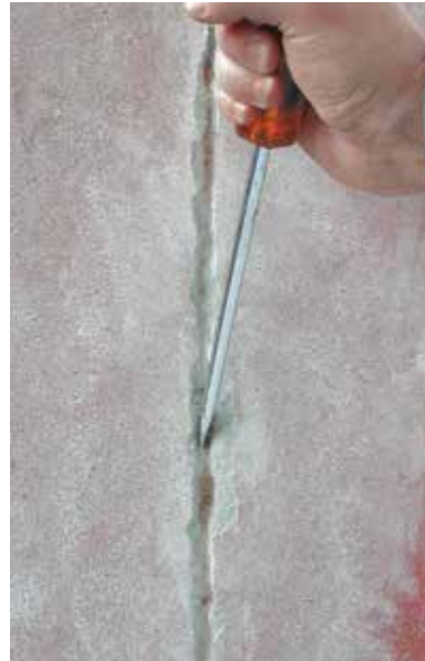
(1) Expanding the crack
